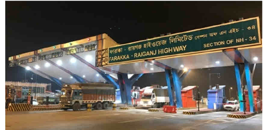
Farakka Raiganj Highway: Toll Plaza at Km 297
