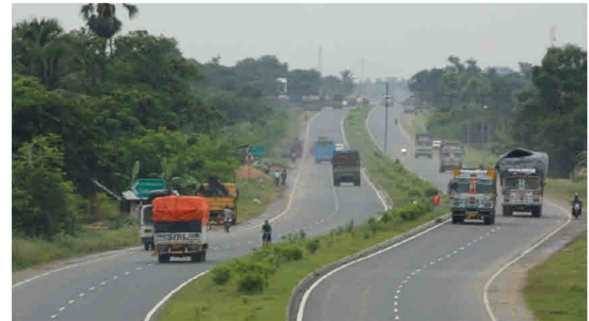
Km 341 (Farakka Raiganj Highway)
