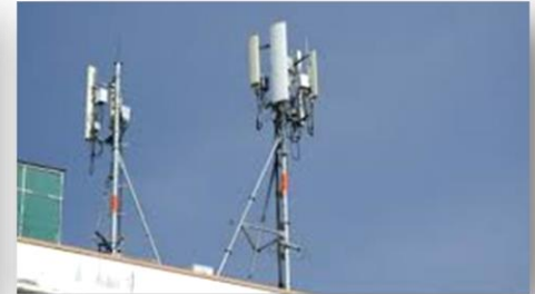
Roof Top Tower
