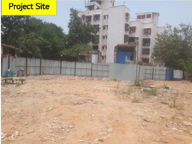
Pota Cabins at Site
