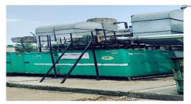
Retrofit Emission Control Device Installation for All DG Sets
