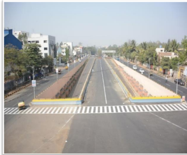
KSB Underpass, Pune
