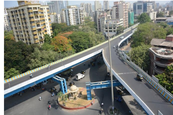
Meenatai Thakre Flyover
