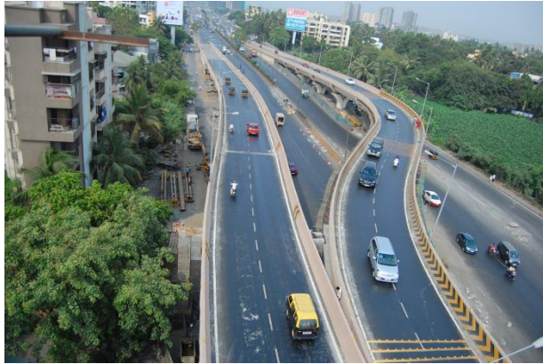
Amar Mahal Flyover
