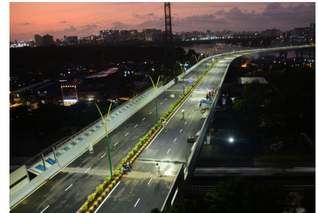
BKC- Chunabhatti Flyover
