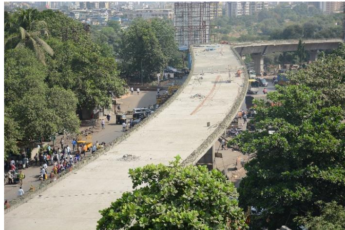
Kalwa Bridge Thane
