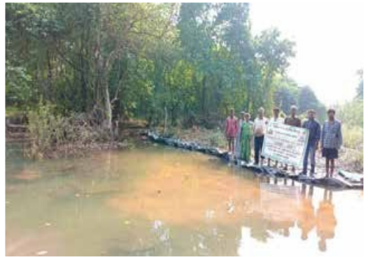
Check Dam: Moravane, Chiplun, Ratnagiri
