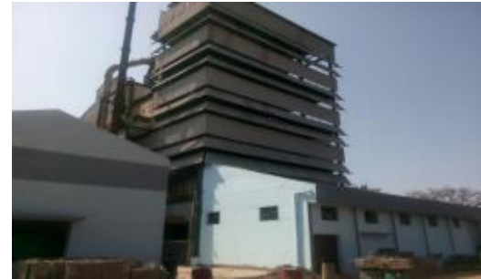
Unit 3 - New Reactive Dyes Plant
