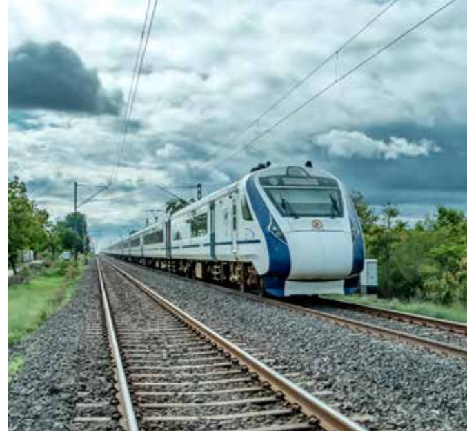
Traction technology and electrification components for semi high speed Indian railways, and Bhopal and Indore Metro
