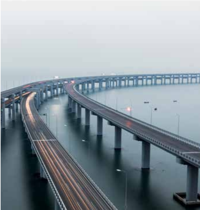
Compact Sub Station (CSS) for one of longest Mumbai Trans Harbor sea link bridge
