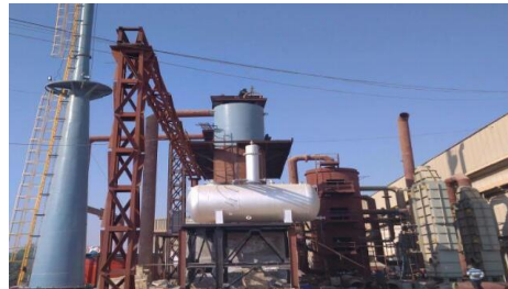
Kisan Phosphates, Haryana: Fertilisers Plant
