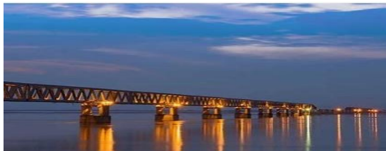
ABB – Compact Power Substations for Bogibeel bridge
