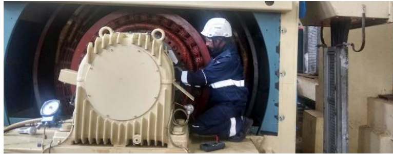
ABB returns power to Kerala after floods take out generator
