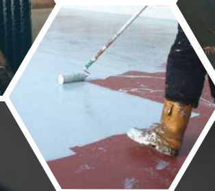
Road Surface Treatment
