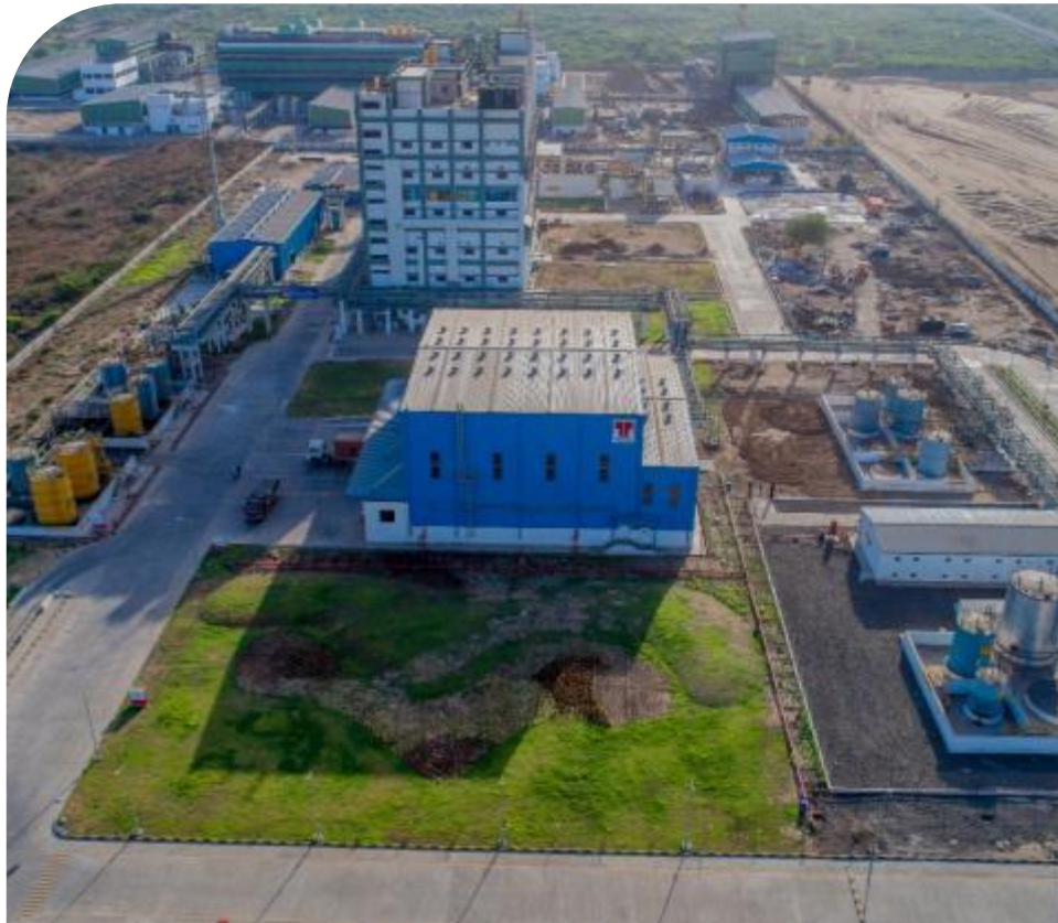
Stabilisation of the Dahej manufacturing facility after the impact of fire incident in June quarter
