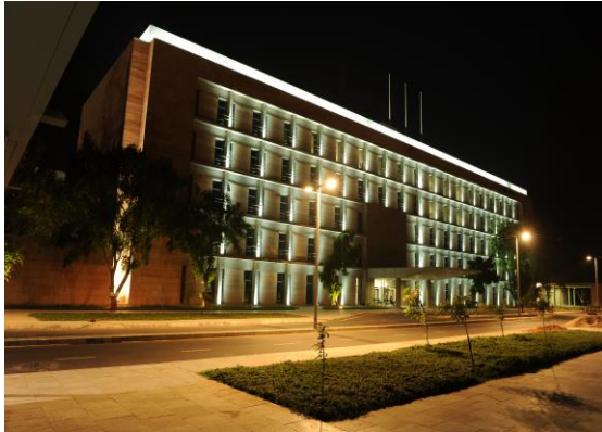
Swarnim Sankul 1 & 2 Construction and interior work
