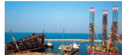
Fabrication Facility, Oman
