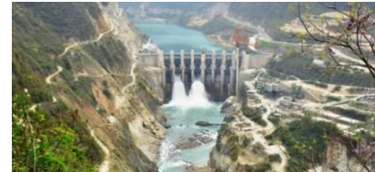
Srinagar Hydro Electric Plant
