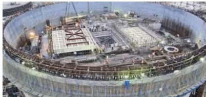
Kakrapar Nuclear Power Plant, Guj
