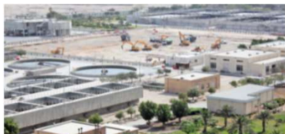
Water Treatment Plant, Doha
