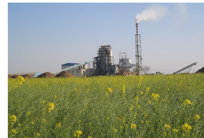
Uniara Power Plant, Rajasthan (India)
