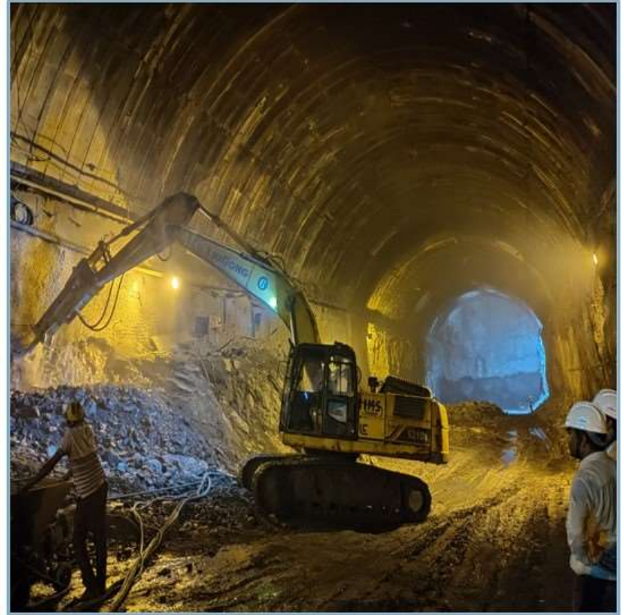
Transformer Hall benching
