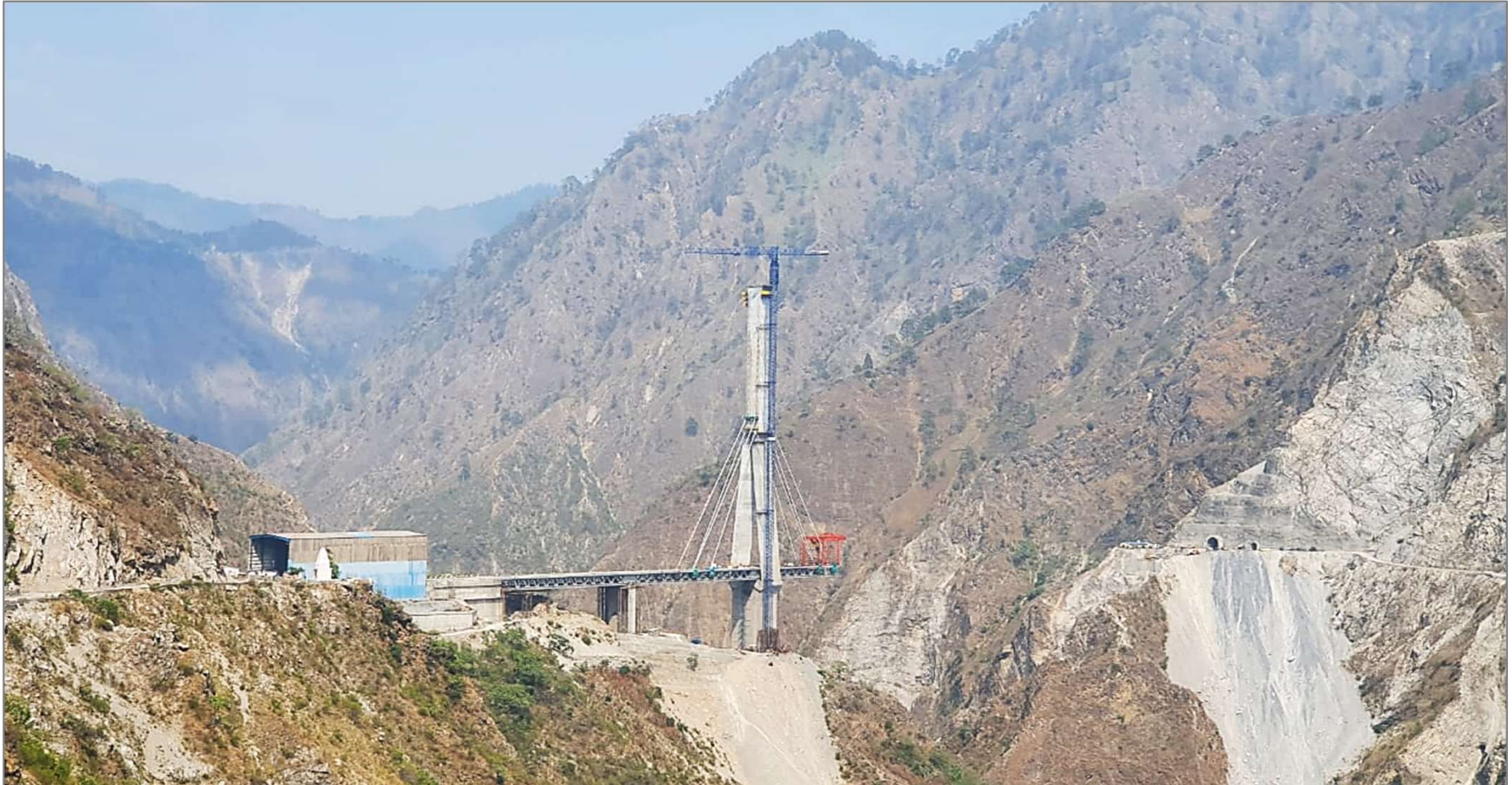
Installation of second cables
