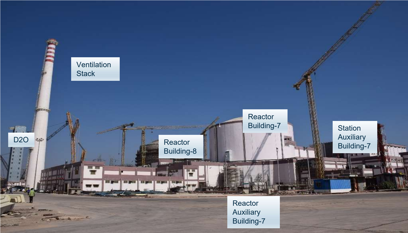
RB-7 & RAB-7, WMP, Ventilation Stack & D2O
