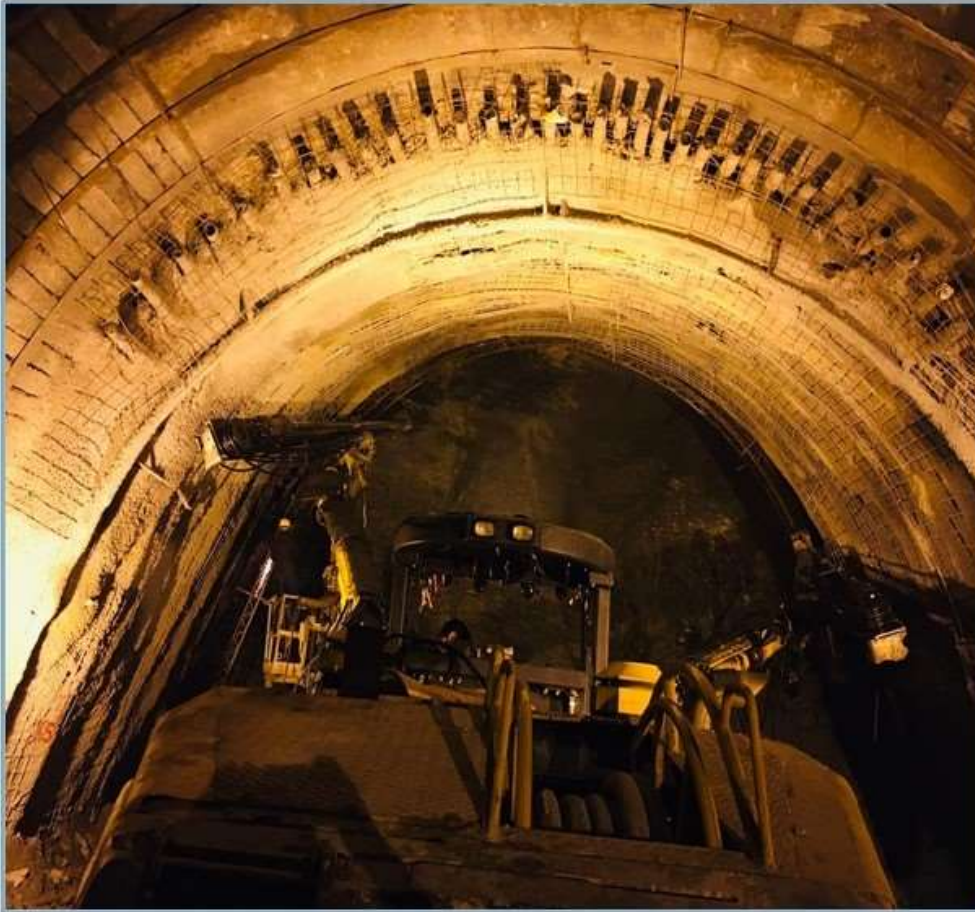
TBM Entry Adit Lattice Girder Fixing
