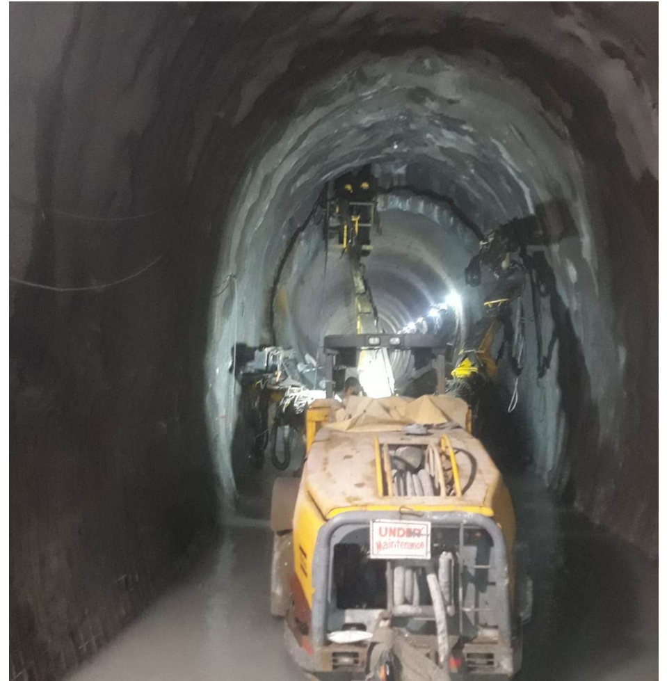
NATM Platform widening
