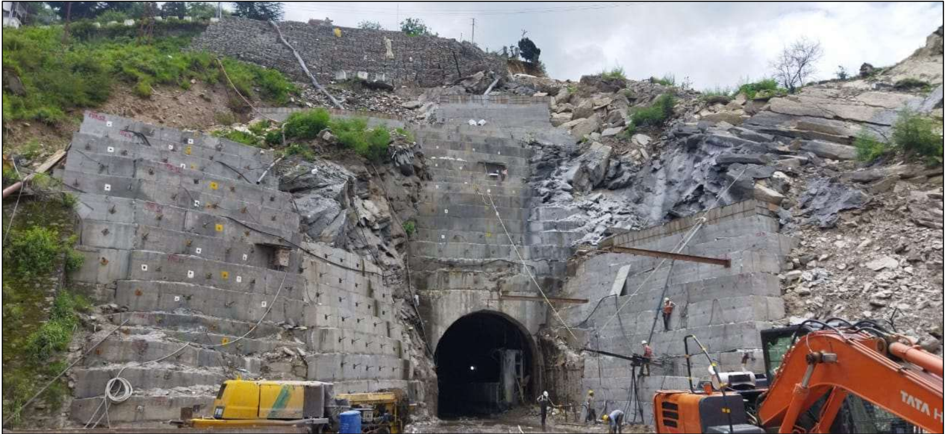
Restoration of TBM Portal
