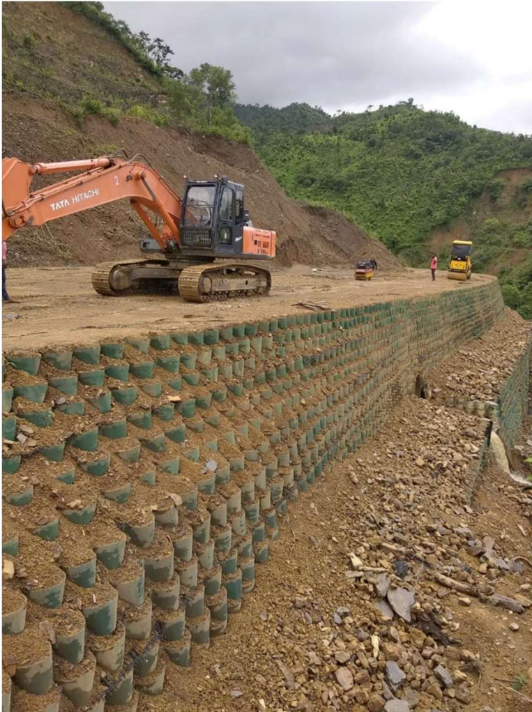
Geo cell works
