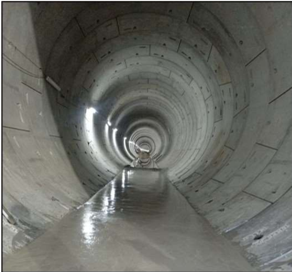
Invert Concrete Completed up to 70 Rm
