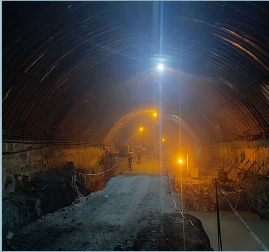
Machine Hall benching
