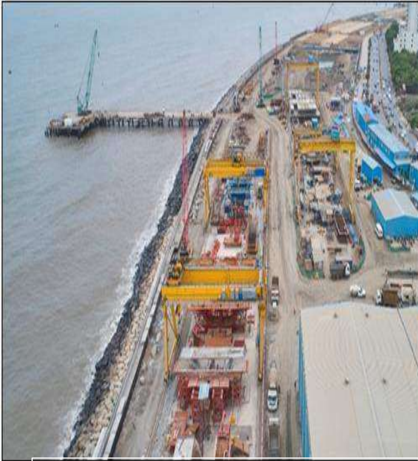
Jetty, Casting yard and seawall
