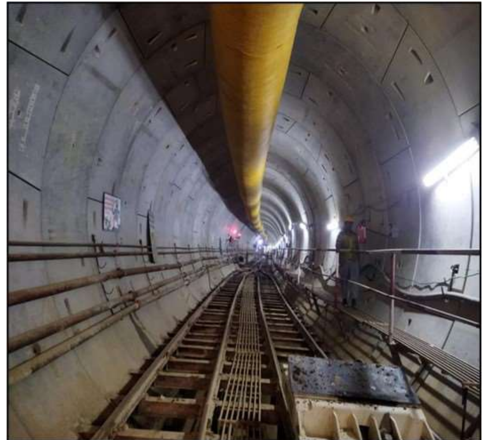
Erection of Segments
