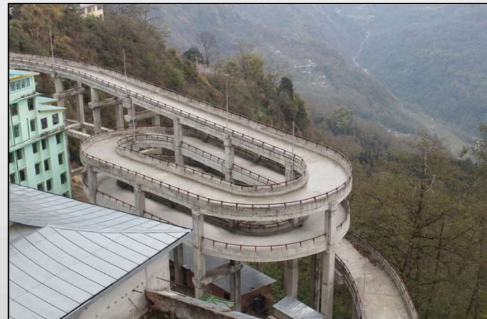
Piling & Civil Works for Gangtok Project
