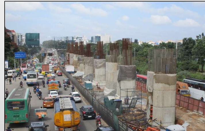
Bangalore Metro Project
