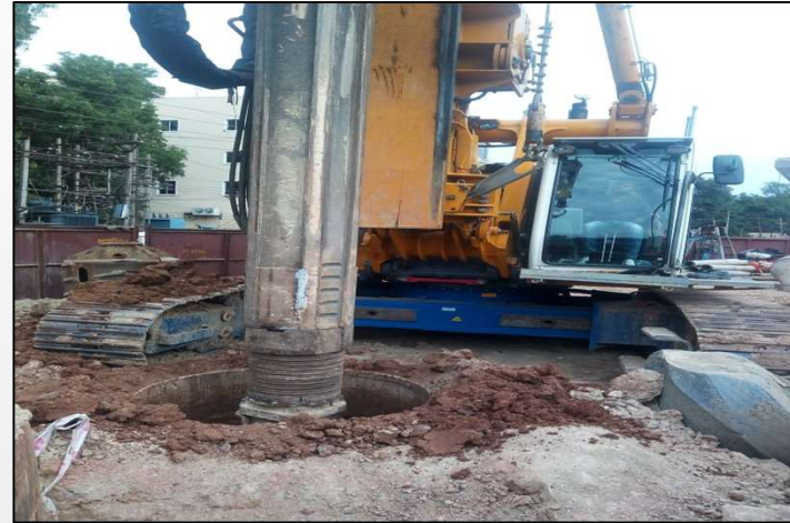
Bangalore Metro Piling Work
