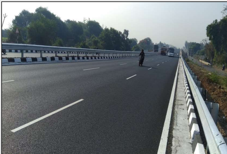
Pune Satara Road Project
