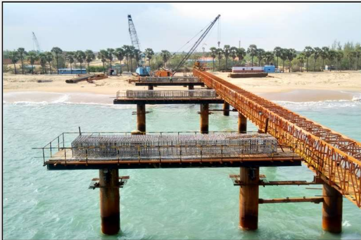
Udangudi Power Project – Piling Work
