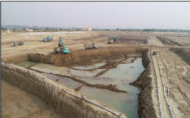
Ground Stabilisation work for Nuclear Power Corporation
