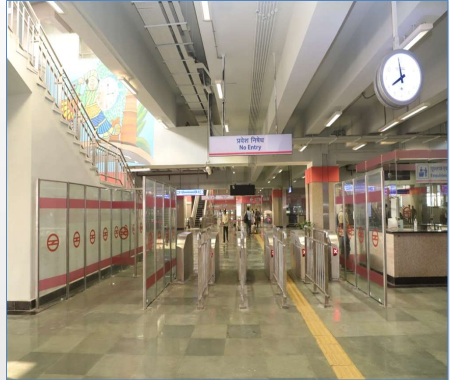
Delhi Metro Elevated Station – CC26
