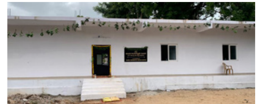
Kitchen & Dining Hall at primary school in Yadadri District
