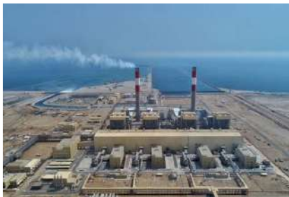
4X660 MW Shuqiaq SSPP, KSA (Completed Project)
