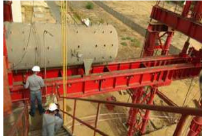
HP Heater Replacement 800 MW, CGPL Mundra 2
