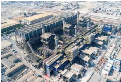
1,800 MW Alba PS5 CCPP, Bahrain (Completed Project)
