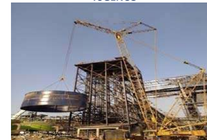
SMS II – Overhead Tank, Dolvi - JSW
