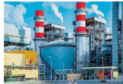
1,516 MW IBRI IPP, SEPCO – 3, Oman (Completed Project)
