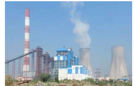
2x660 Mw STPS, Suratgrah - RRVUNL
