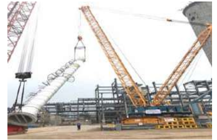
Urea Reactor Tank Installation At Ramagaundam, Telangana
