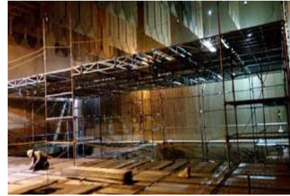
Cuplock Scaffolding Erection 800 MW, Mundra
