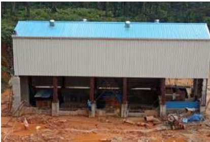
Implementation of Hydro Electric Project (2MW/5.14 Mu)-KSEB
