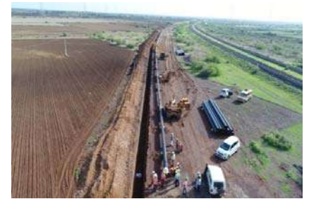
Lowering of pipe at Mundra to Kandla pipeline project-90 KM, Adani
