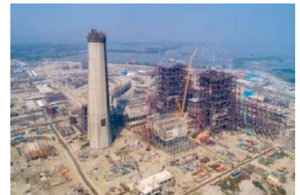
2X660 MW at Rampal, Maitree, Bangladesh-BIFPCL
