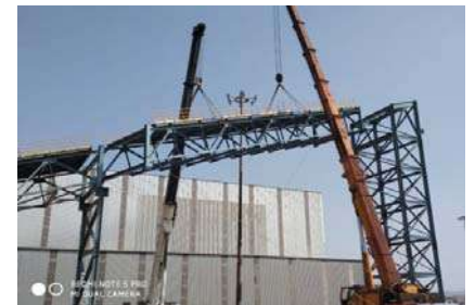
Erection of P&N Gallery at Bellary, JSW
