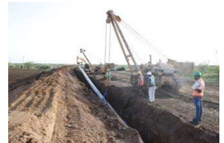
Lowering of Pipe Section, Mundra, Adani
