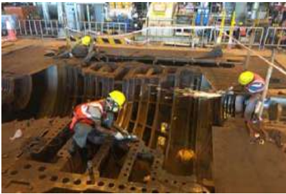
Main Turbine Overhauling, 660 MW, Kawai
