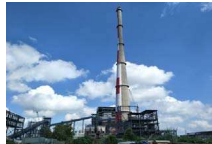
1x660 MW Harduaganj TPS, UPRVUNL
