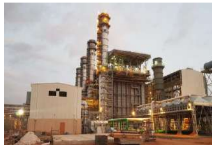
1,390 MW Waad Al Shamal ISCCPP, GE, KSA
