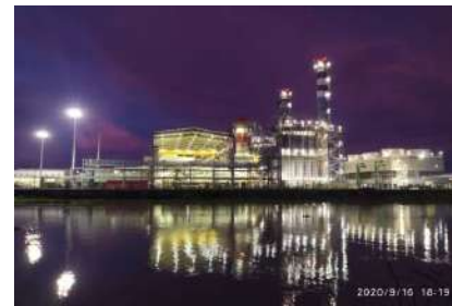
220 MW (GAS) / 212 MW, (HSD) CCPP, Bisho Infra, Bangladesh
