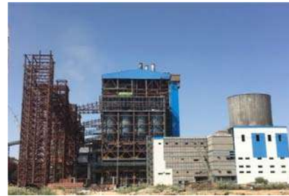
2x660 MW Suratgarh STPP, RRVUNL
