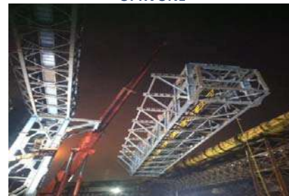
Utility Corridor, Gallery Erection, Dolvi, JSW
