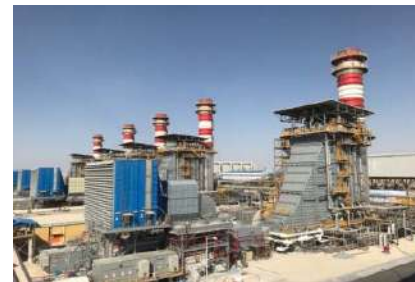
1,519 MW Fadhili CHPP, Doosan, KSA
