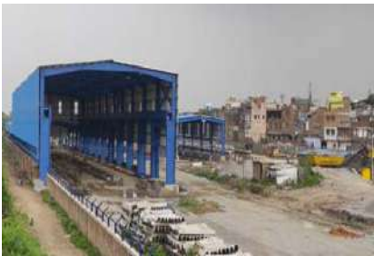
MEMU Shed at Kanpur-RVNL
