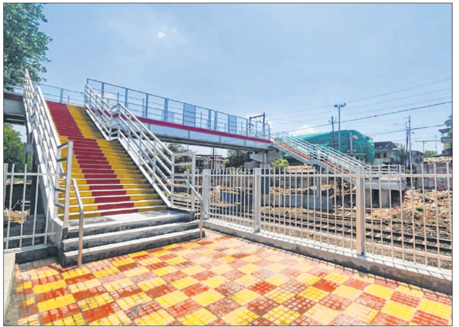
MRVC has commissioned a new foot over bridge at the Kalyan end of Ambivali station. The 23mt long and 4mt wide bridge will cater to nearly 30,000 daily footfalls. The project cost was ₹1.4 crore.
