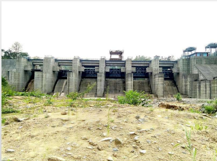
New Hydro Dam Umtru
