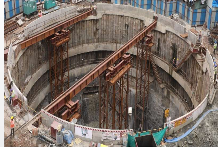
Diaphragm Walling at Mumbai Metro Line 3
