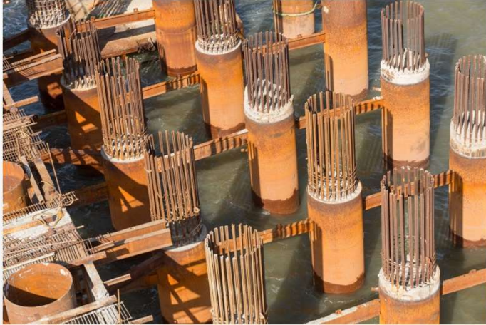
Marine Piling for Mumbai Port Project
