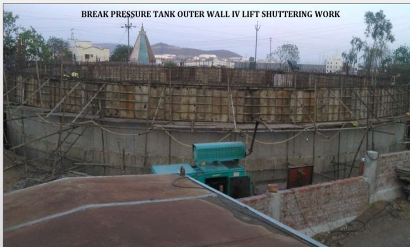
Break pressure tank work in progress, Bhama, Pune
