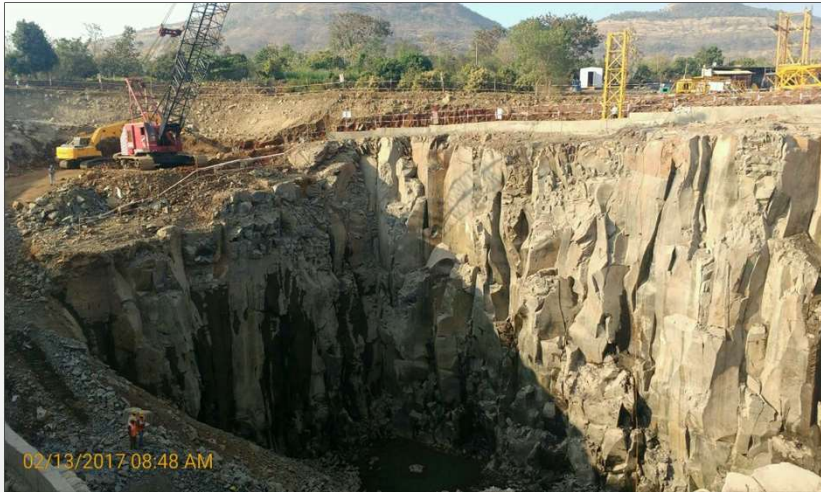
Bhama Ashed Water Supply Project
