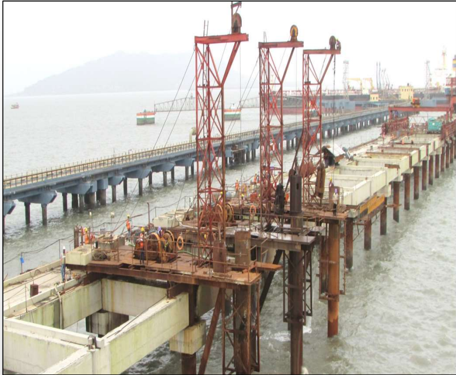
Construction Work at Mumbai Port Trust
