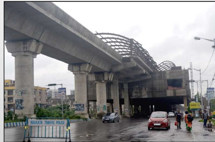
Kolkata Metro Station
