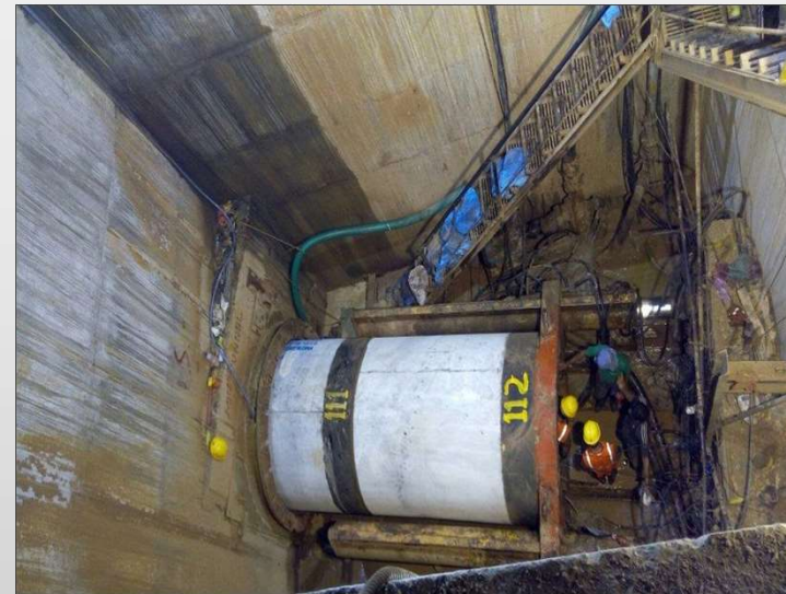
VMSS – Micro Tunneling Vadodara
