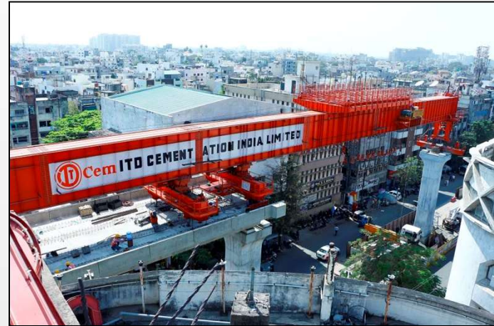
Nagpur Metro Elevated Project
