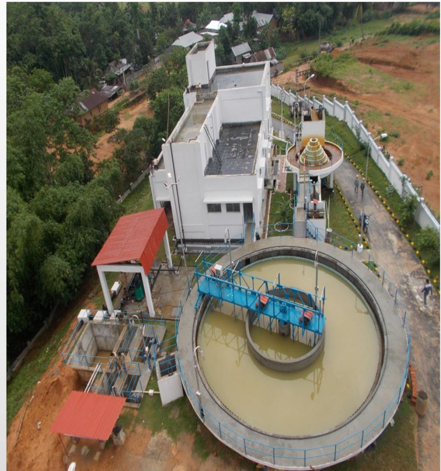
Agartala WTP project
