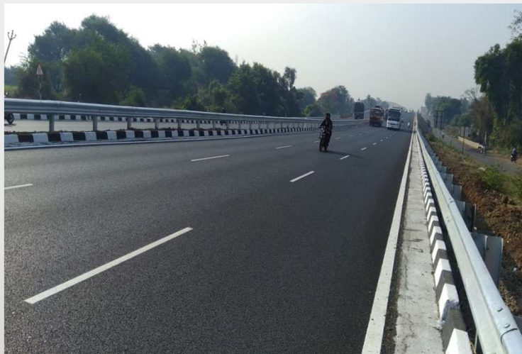
Pune Satara Road Project
