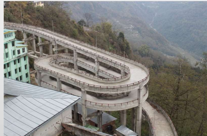
Piling & Civil Works for Gangtok Project
