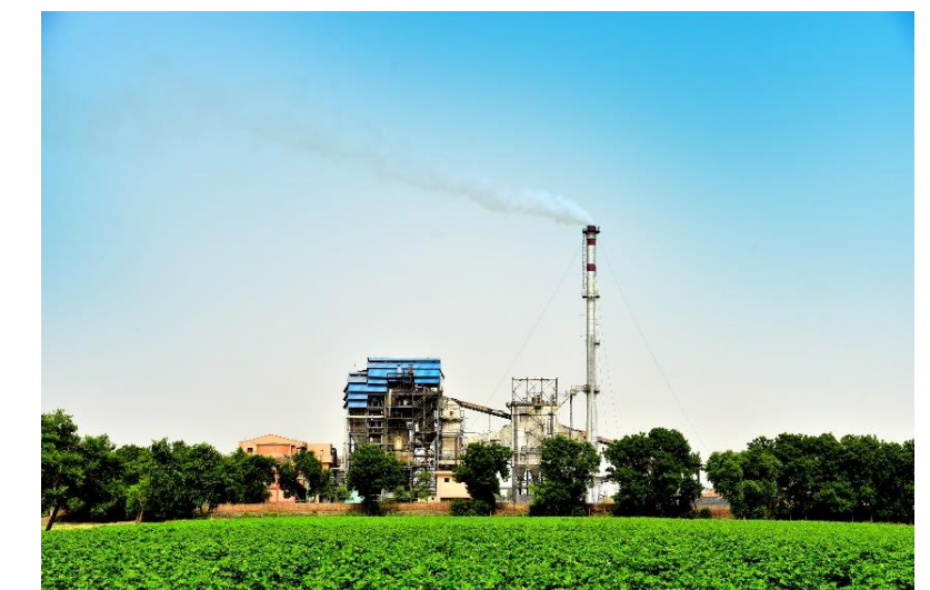
Padampur Power Plant, Rajasthan (India)
