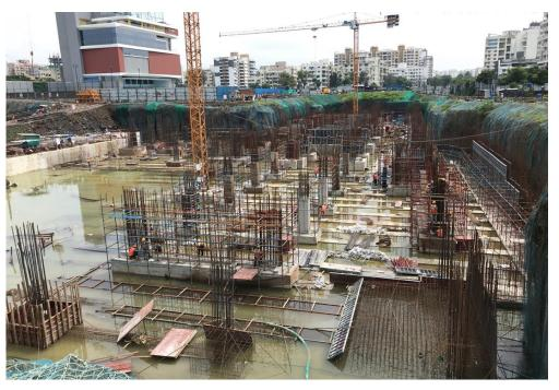
Excavation is complete, foundation & retaining wall work is in progress
