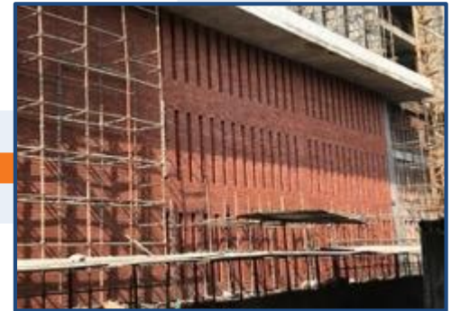
September 2019 Structure completed
