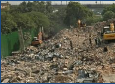
November 2018 Existing building demolished; construction started
