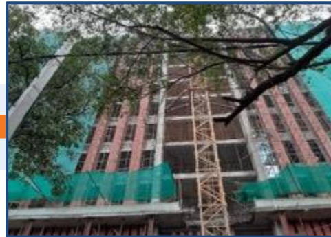
January 2020 Façade & Services installation
