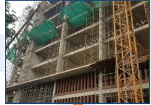
June 2019 Structure completed upto L6
