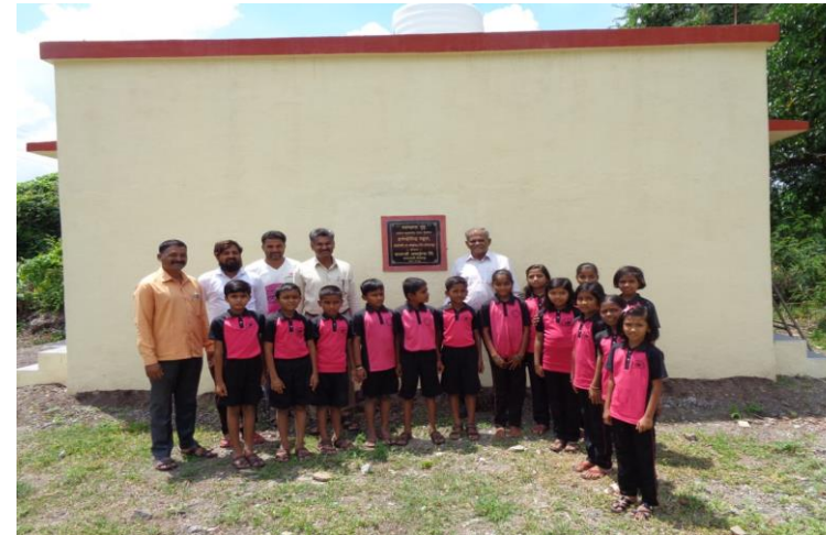
Constructed Ladies And Gents Toilet Block At Innovative School Ankoli Taluka Mohol District Solapur Dt 03.09.2022
