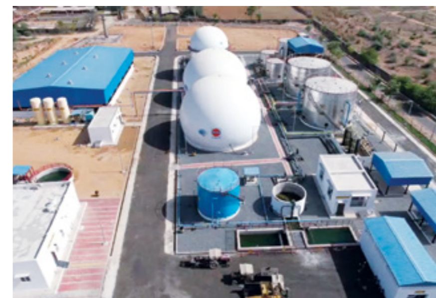
CBG plant at Hingonia, Jaipur
