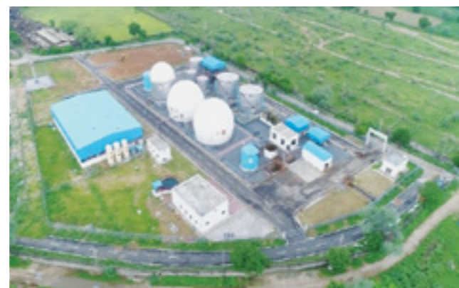
100 TPD Compressed Biogas Plant at Hingonia, Jaipur
