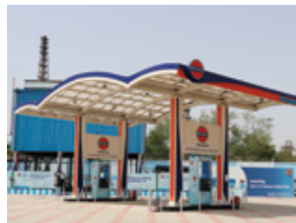
Hydrogen fuel station at Gujarat Refinery
