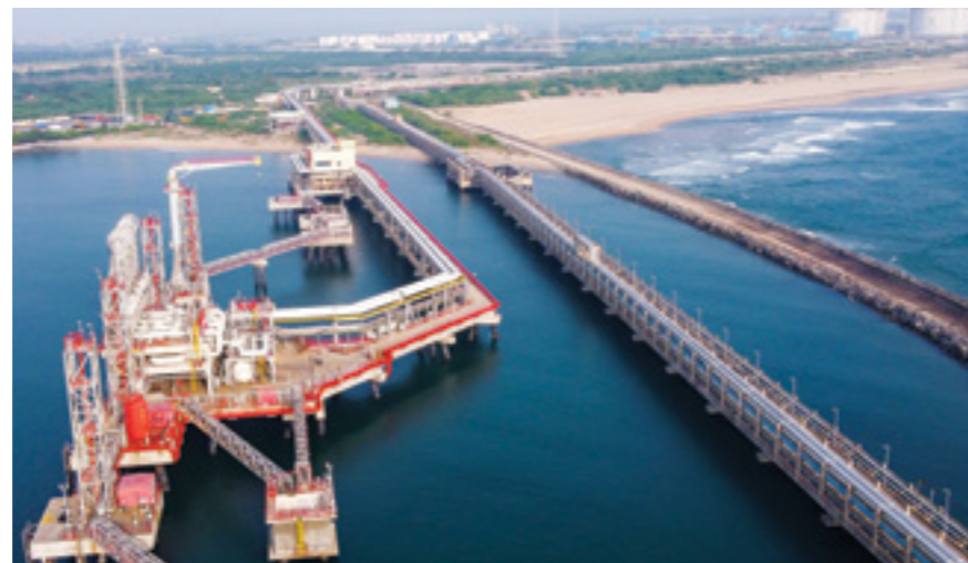
Marine facilities for LNG unloading at Ennore, Tamil Nadu
