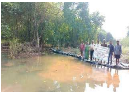
Check Dam: Moravane, Chiplun, Ratnagiri
