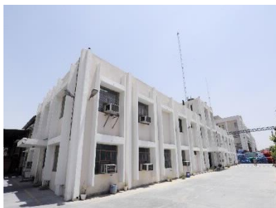
RFL I & II- Bahadurgarh
