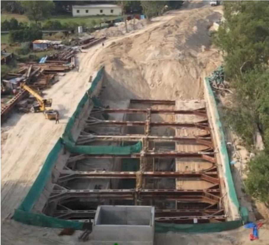
Cut & Cover Roof slab
