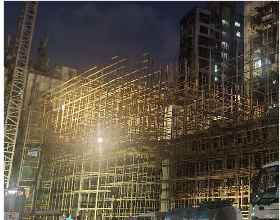
Ancillary Building works
