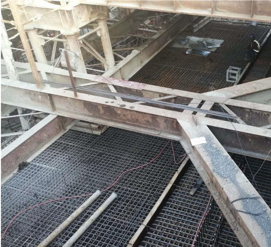
Station works – Concourse Slab
