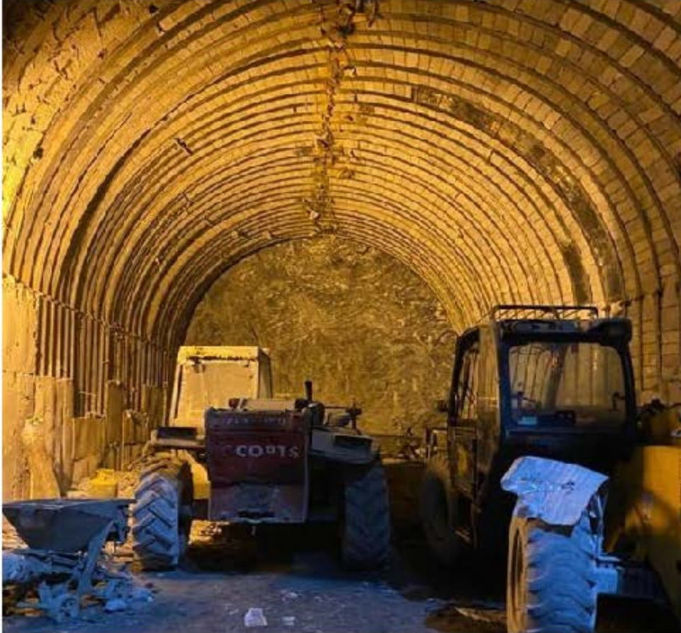
Horizontal Penstock Excavation
