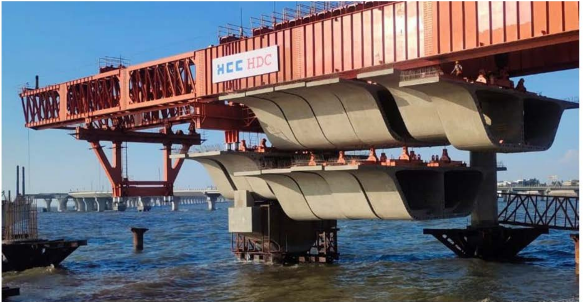
Main Bridge - Segment Launching
