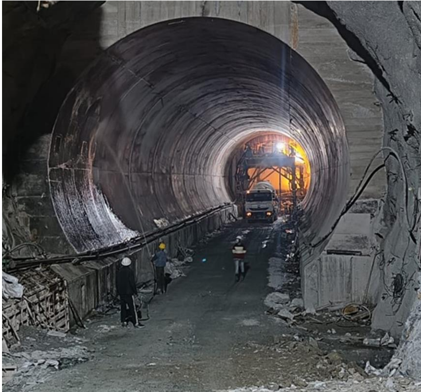
HRT Overt lining
