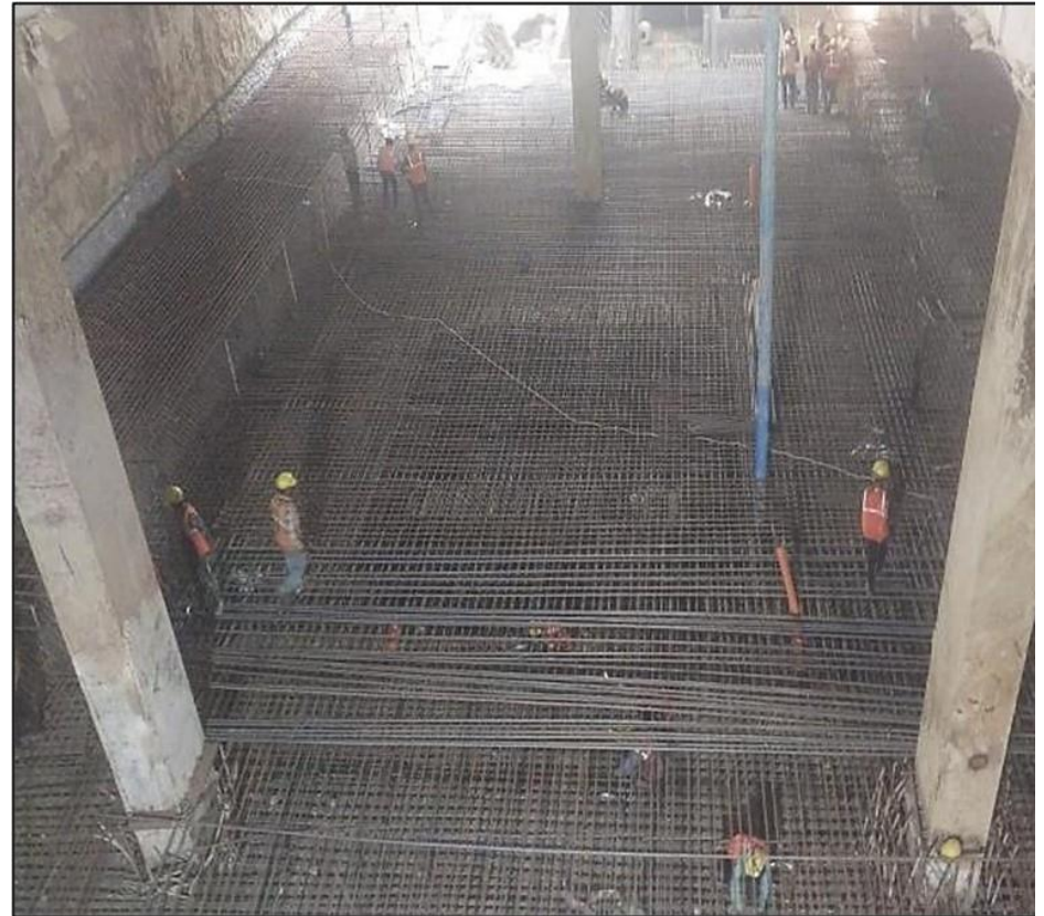
Station Base slab works Grid 5-8
