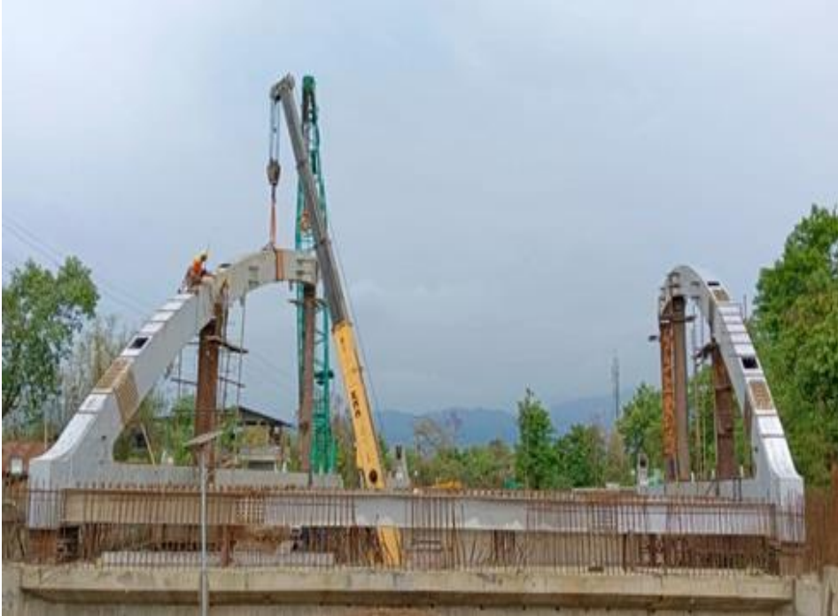
Bow string girder erection @ Bridge 5+411
