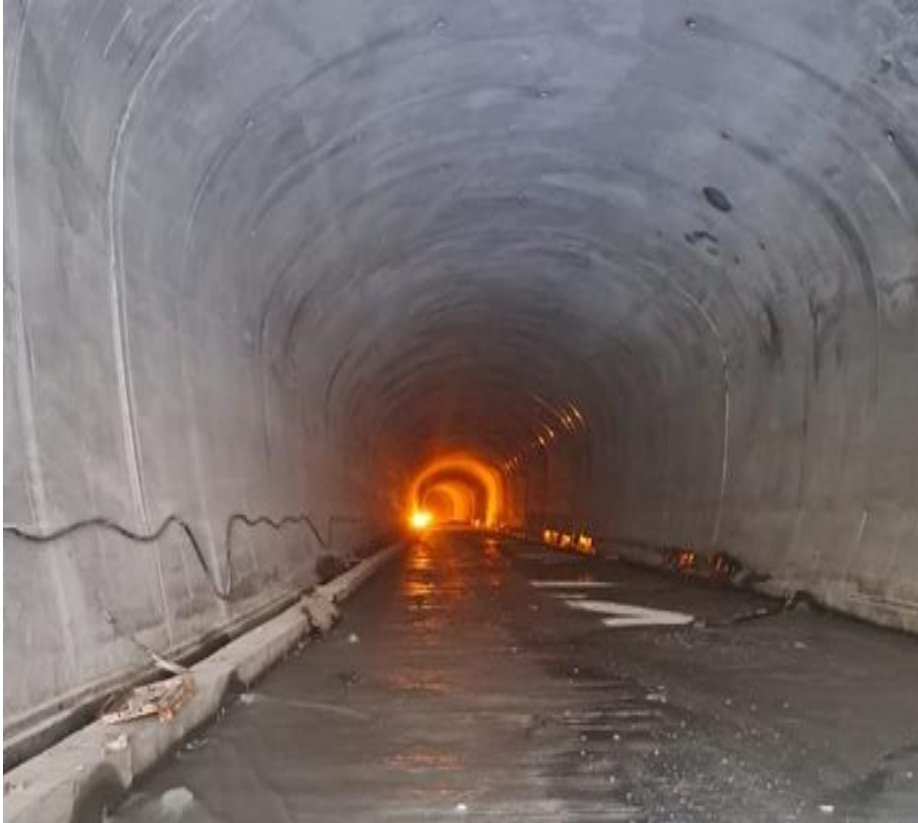
Tunnel invert lining
