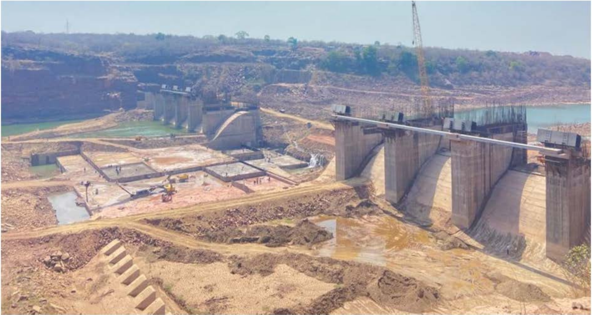
Dam and Tunnel works are progressing well
