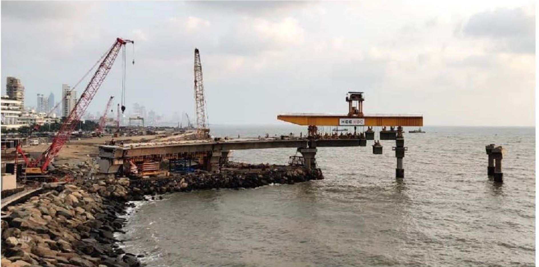
Arm – 2 Segment Launching
