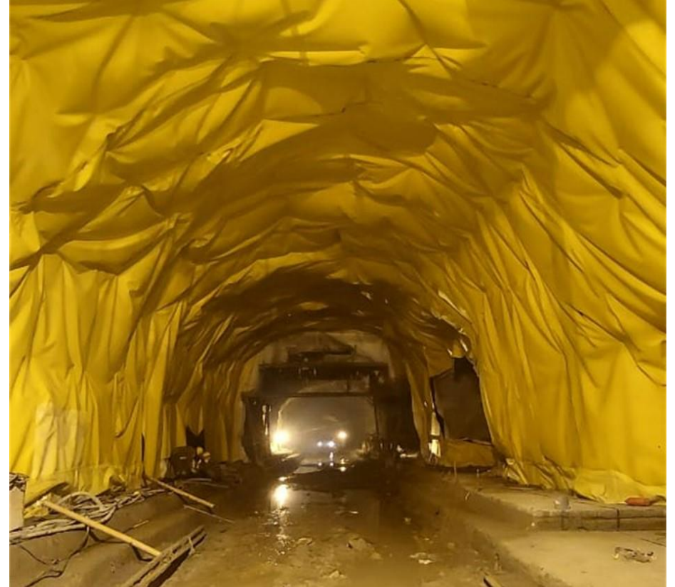
Escape Tunnel Layby Water Proofing Membrane fixing
