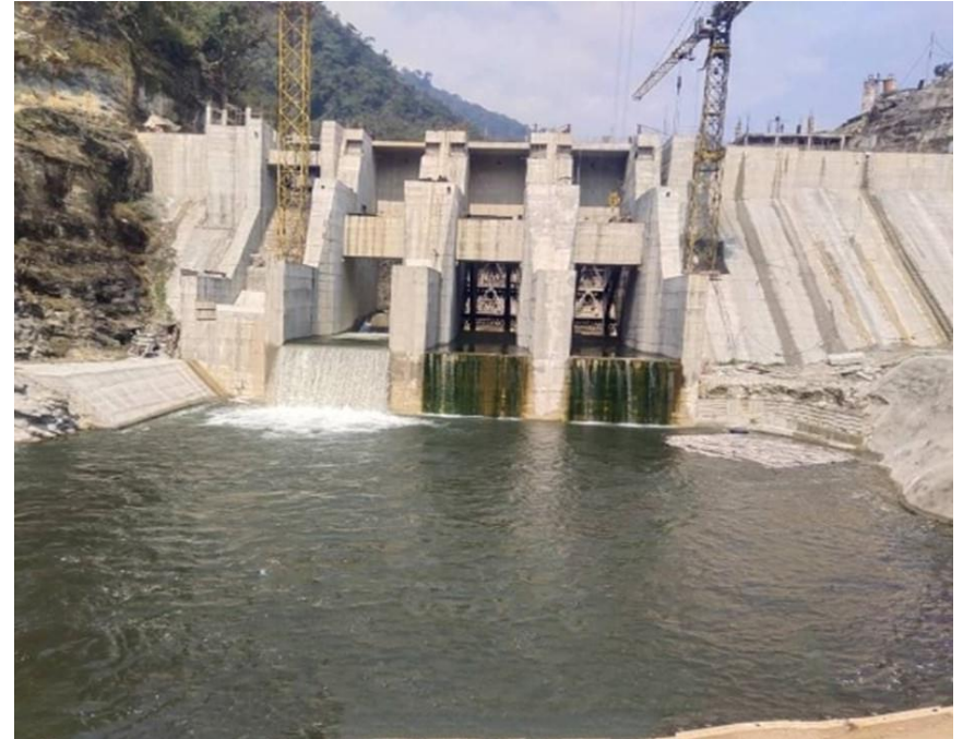
Dam works – River diverted through Radial gates
