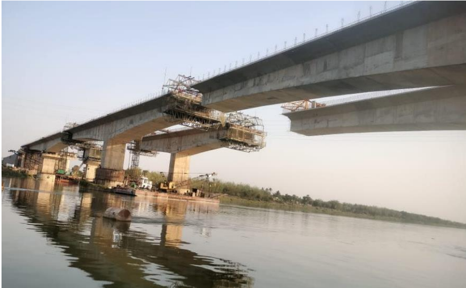
Bhagirathi bridge super structure works
