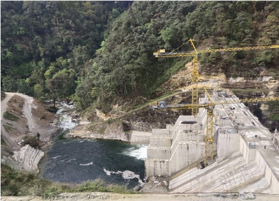
Dam works – River diverted through Radial gates
