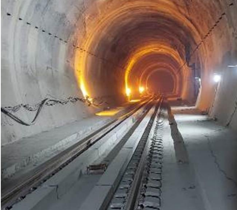
Main Tunnel with BLT
