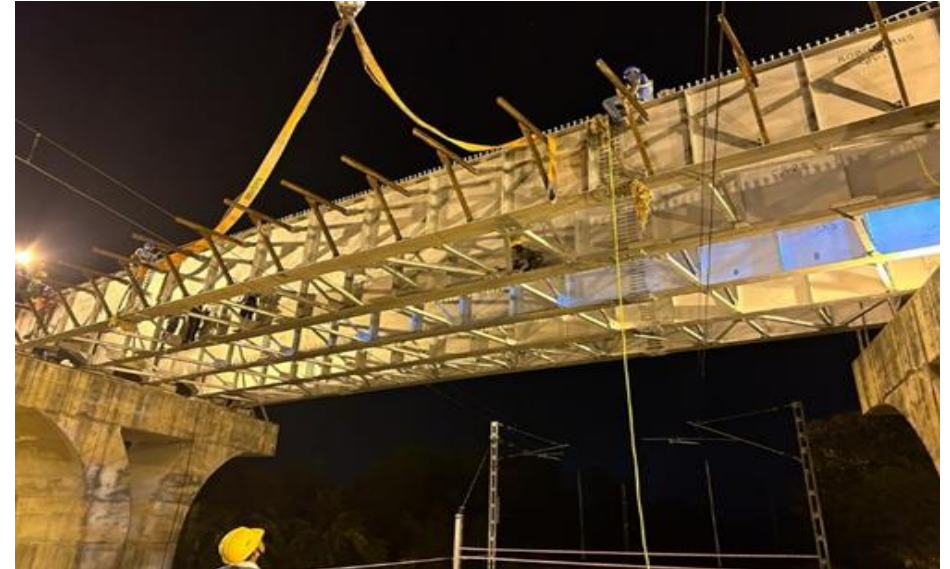
ROB at Ch 192 (RHS): Steel girder erection work in progress
