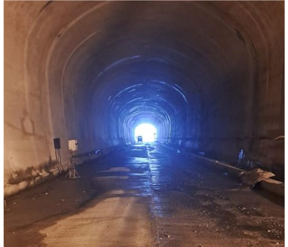
Tunnel Overt lining
