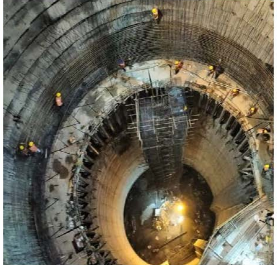
Downstream Surge Shaft Lining
