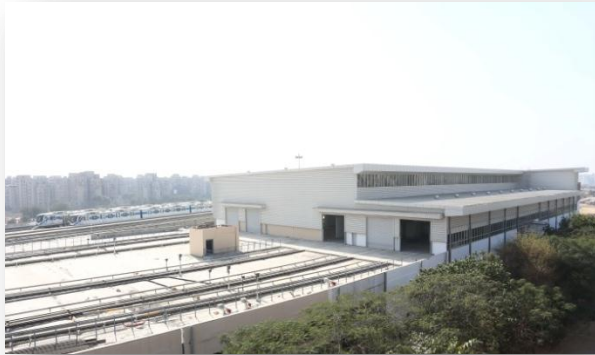
IL&FS Transportation Network Ltd (Gurgaon, Haryana)
