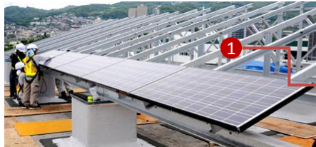
Solar Panel Structural Support (IS277 GP550,550GSM - GP)
