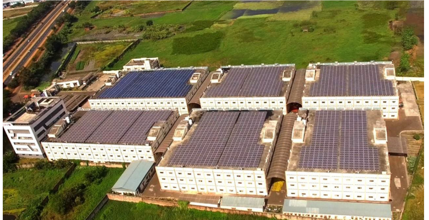
Rooftop solar power plant at Dankuni unit
