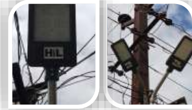
Installed LED streetlights on the way to timmapur village
