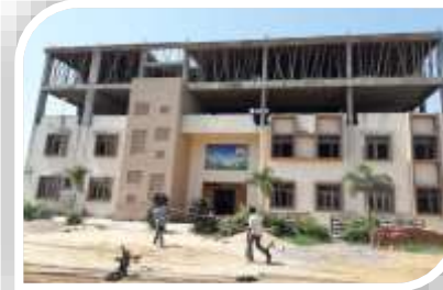
Provided AAC Blocks to construct floor to govt. School
