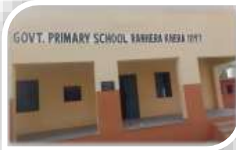
Renovation of Primary Govt School at Faridabad
