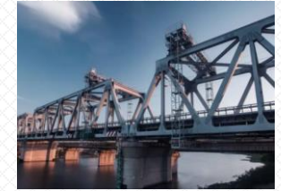
Heavy Steel Structures
