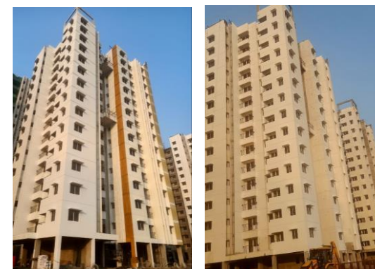
External painting Done – Custer A & B
