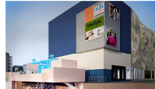
Underground 132 kV SS at 'Quest Mall'
