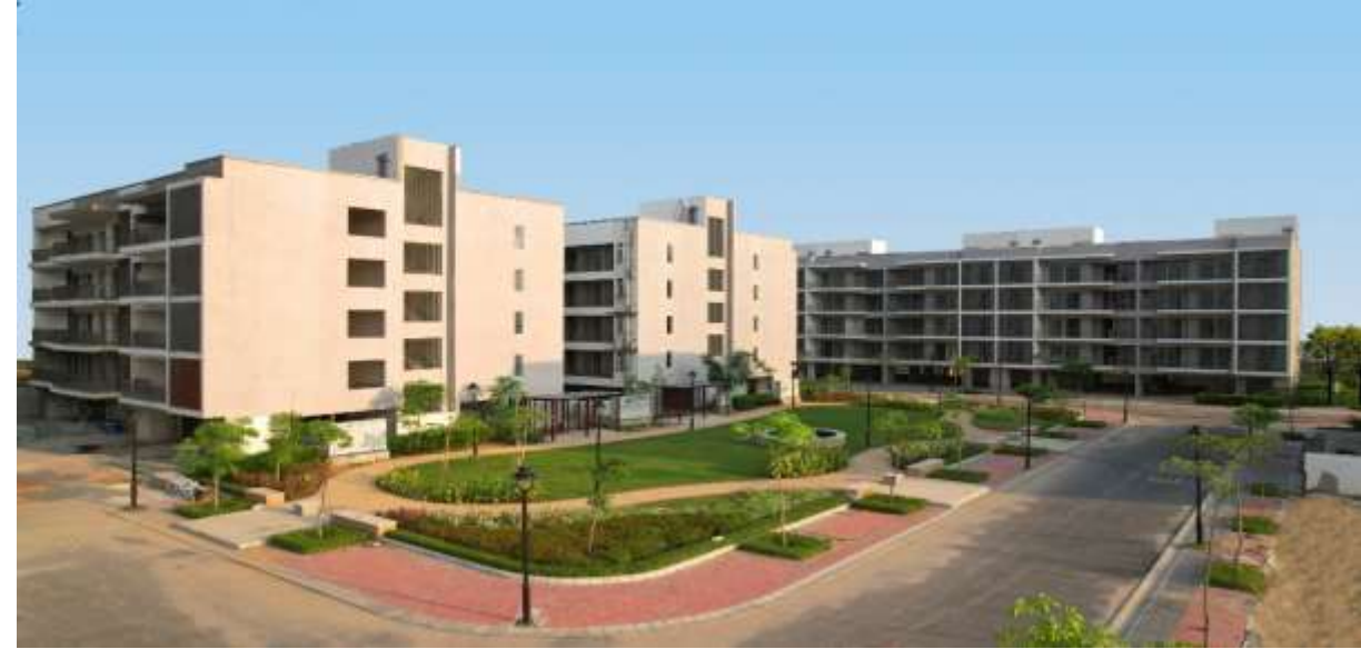
Garden city Floors, New Gurgaon
