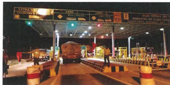
Development & Operation of Bikaner-Suratgarh Section of NH-62 (earlier NH-15) in the state of Rajasthan
