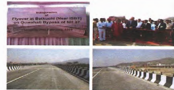
Construction of 2 lane flyover on Guwahati Bypass of NH-115 (earlier NH-37) in the state of Assam
