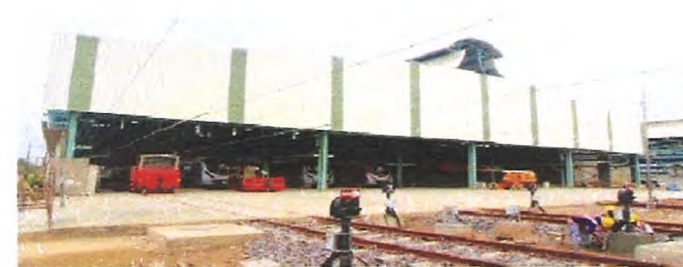
Construction of Metro rail depot, Kalindi Kunj, New Delhi
