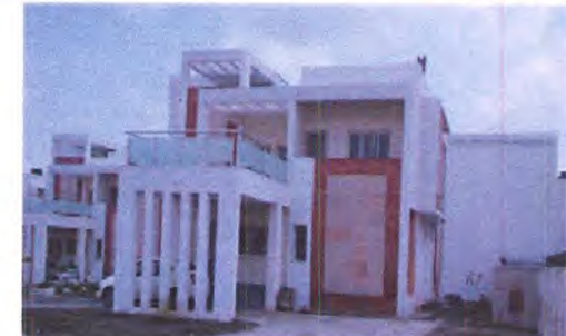
Construction of Director, Dean Bungalow, QIP Centre & Accommodation for School of Planning & Architecture at Bhopal
