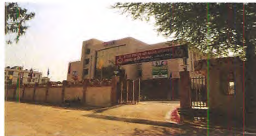
Construction of Police station & Residential Quarters, Hari Nagar, Delhi for MHA, Delhi Police through RITES Ltd.
