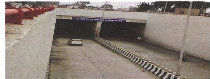
Construction of RUB at Badli, New Delhi
