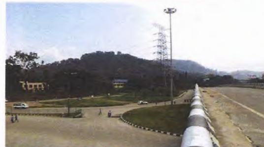
Widening & Strengthening of existing National Highway from 2 lane to 4 lane of Sonapur to Guwahati section of NH-115 (earlier NH 37)
