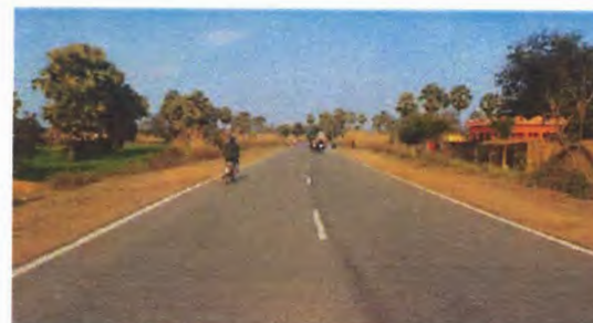
Upgradation of roads and bridges of Shivganj-Rafiganj-Goh-Uphara-Devkund-Baidrabad Road (SH-68, in the state of Bihar)
