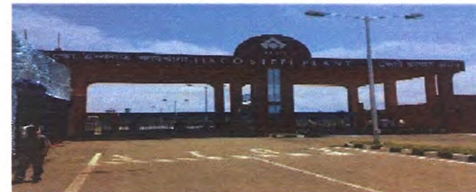
Approach Road 2 lane from GT Road at Neamatpur to Burnpur, West Bengal
