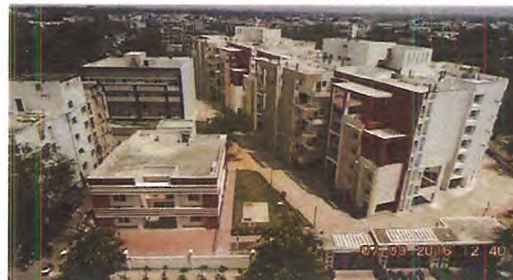
Construction of 92 flats at Mahadev Towers, Bhopal for MP Housing & Infrastructure Development Board
