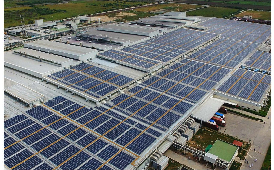
Honda Motorcycle and Scooter India Manesar, Tapukera, Vithalapur, Narsapura 25 MW rooftop solar project Largest rooftop implementation by Bosch
