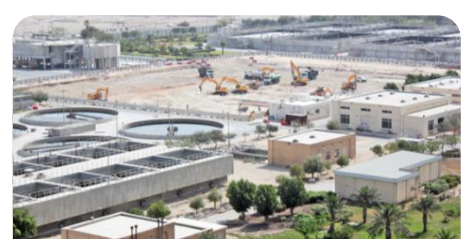
Water Treatment Plant, Doha
