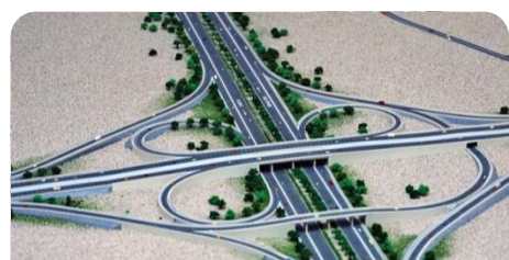
Sheikh Khalifa Interchange, UAE
