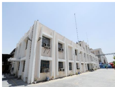
RFL I & II- Bahadurgarh
