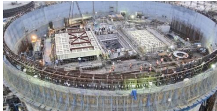
Kakrapar Nuclear Power Plant, Guj
