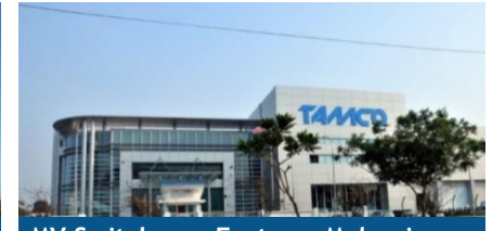
MV Switchgear Factory, Malaysia
