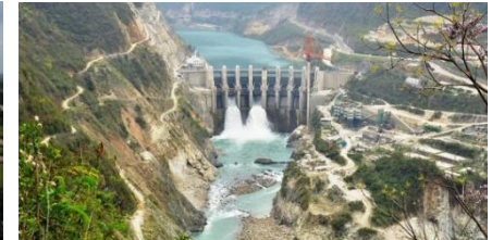
Srinagar Hydro Electric Plant
