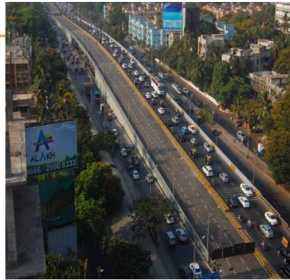
Kherwadi Flyover, Mumbai
