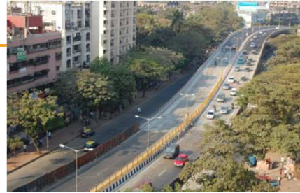
Flyover at Hindmata
