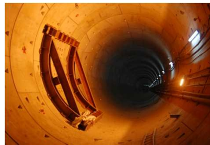
DMRC CC-24 Tunnel
