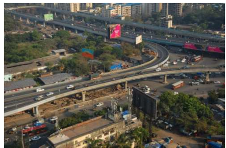
Flyover at Kapurbawadi
