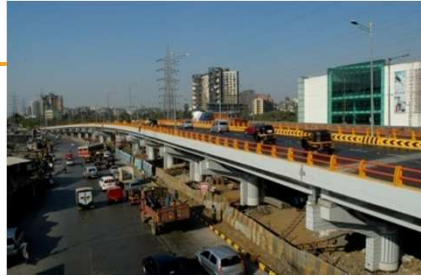
Flyover at Dindoshi, Mumbai
