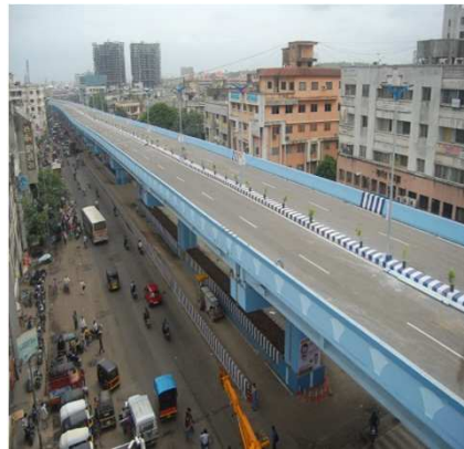
Dhankawadi Flyover, Pune
