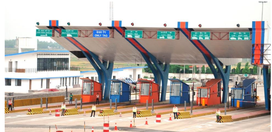
Package 3 Toll Plaza at Km 206
