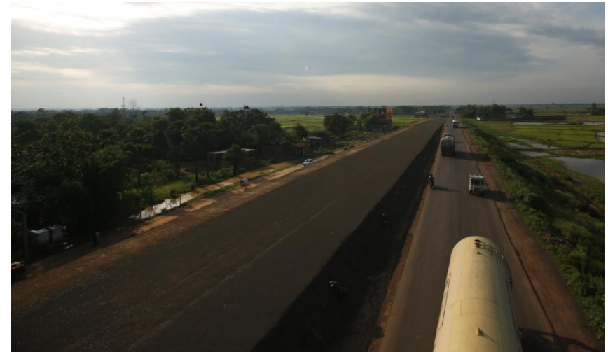
Construction underway at Package 4
