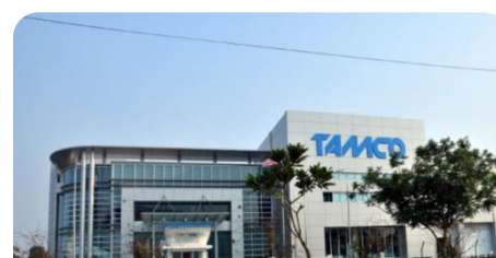
MV Switchgear Factory, Malaysia
