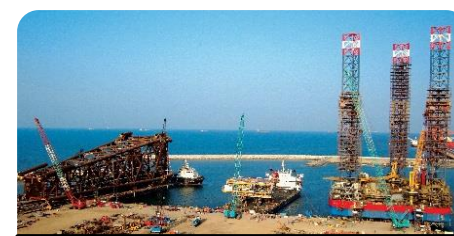
Fabrication Facility, Oman
