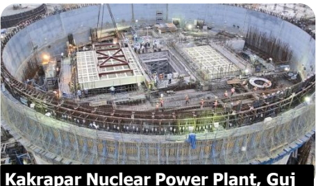
Kakrapar Nuclear Power Plant, Guj
