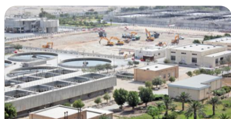
Water Treatment Plant, Doha
