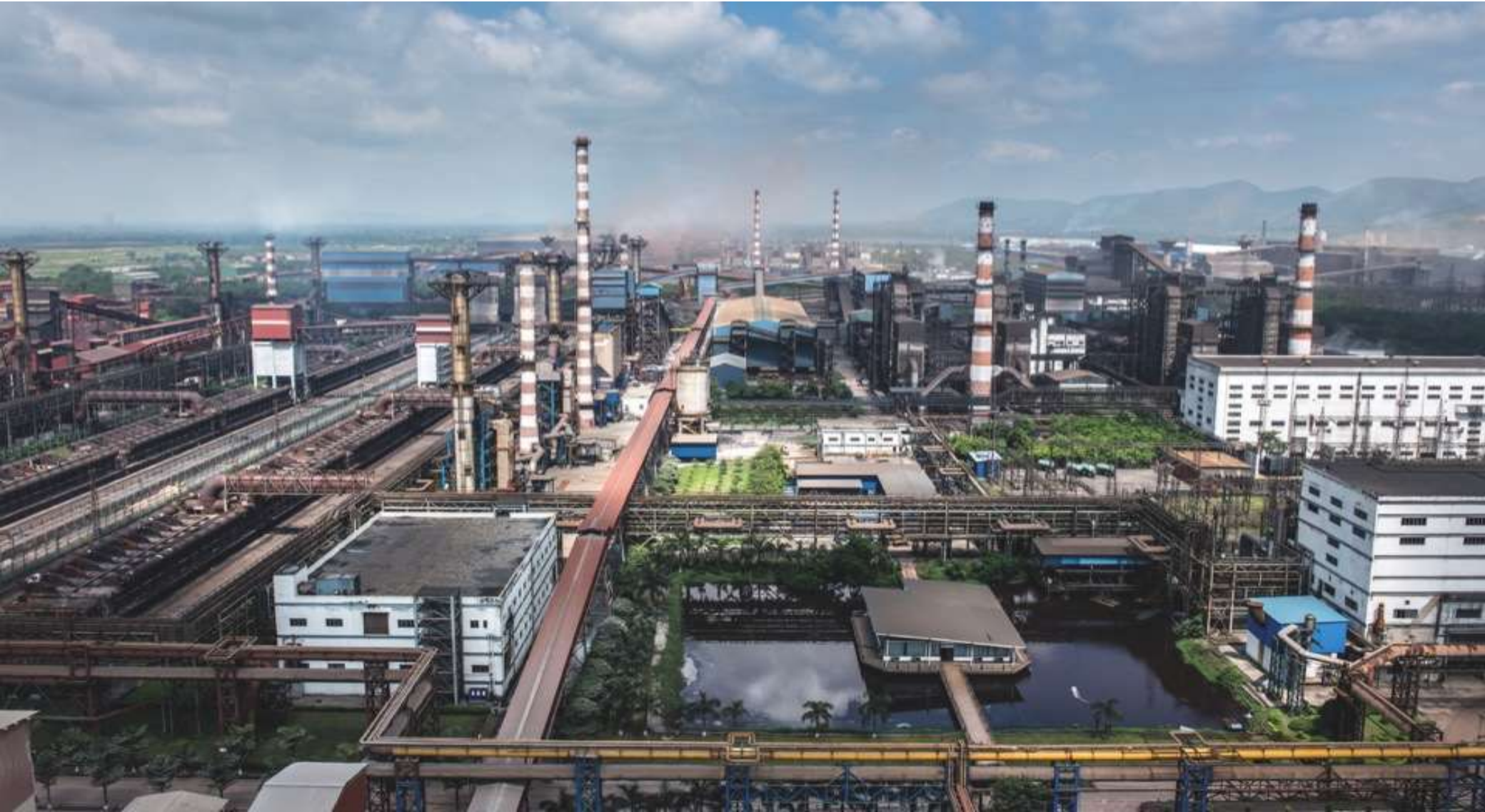
Aerial View of Raigarh Plant
