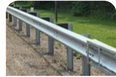
Metal Beam Crash Barrier
