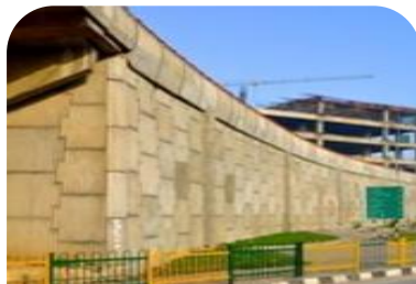
Reinforced Earth Walls
