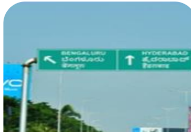
Overhead Cantilevers and Gantries
