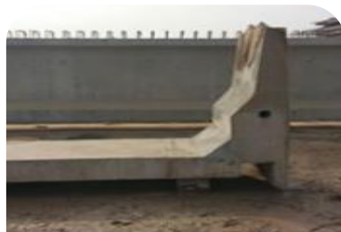
Fabricated Casting Panels and Moulds
