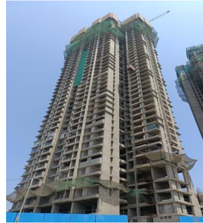
Tower (A) 37 th Floor Slab Completed
