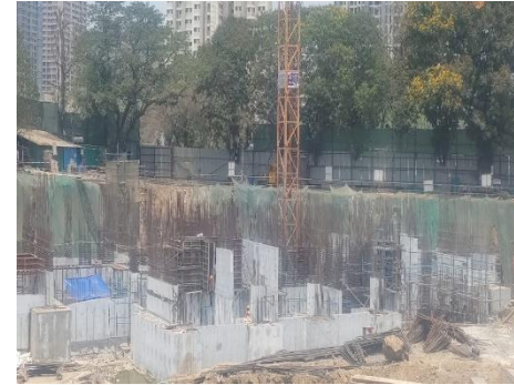
Tower (C) Plinth slab work in progress
