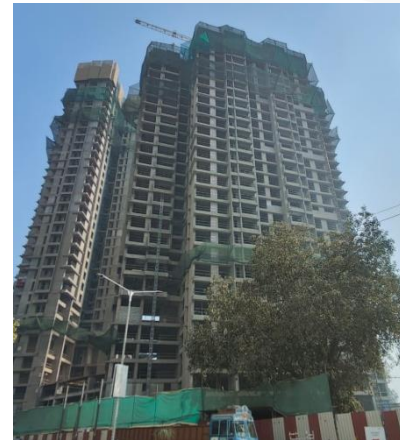
Tower (B) 29 th Floor Slab Completed
