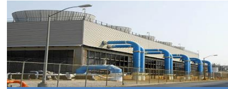
Infrastructure Construction (Civil)
