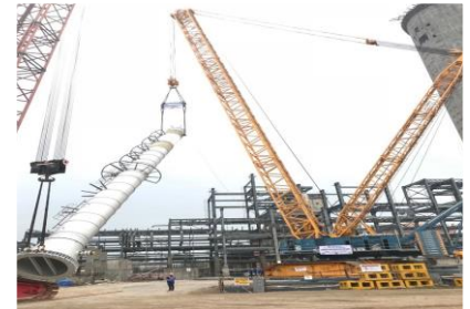
UREA REACTOR TANK INSTALLATION AT RAMAGAUNDAM, TELANGANA
