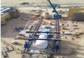
1519 MW FADHILI CCPP, SAUDI ARABIA GTG,STG & BOP INSTALLATION
