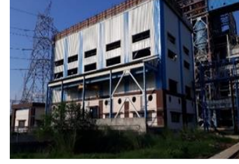
1X500MW, FGUTP, CIVIL, STRUCTURAL AND ARCHITECTURAL WORK FOR BTP, BOP & CHP, UNCHAHAH, NBPPL
