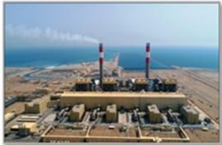
2X640 MW SHUQAIQ THERMAL POWER PLANT, SAUDI ARABIA (COMPLETED)
