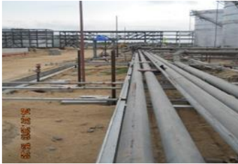
3X366 MW CCPP, CIVIL, STRUCT. & ARCH. WORK, IOCL PARADIP, BHEL
