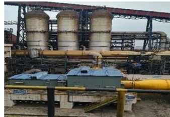
BLAST FURNACE, STEEL PLANT WORK, JSPL, ANGUL
