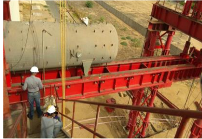
HP HEATER REPLACEMENT 800MW ,CGPL MUNDRA2
