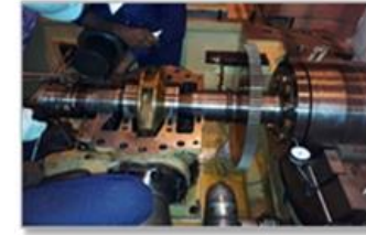
228MW, STEAMTURBINE, SABIYA, KUWAIT, MAIN OIL PUMP OVERHAULING
