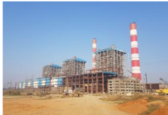
3X660 MW ,BOILER, ESP,CP, STRUCTURE & STG, NABINAGAR, BHEL
