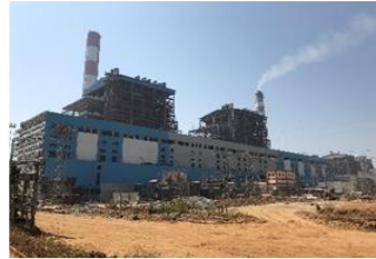
2X660 MW IBTPS, STRUCTURE & STG, BANHARPALLI, BHEL
