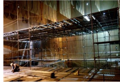
CUPLOCK SCAFFOLDING ERECTION 800MW,MUNDRA
