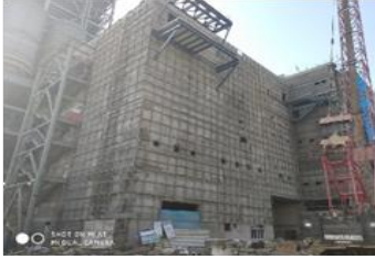
1X800 MW TPSS, CIVIL, STRUCTURAL AND ARCHITECTURAL WORK UNIT-12, KOTHAGUDEM, BHEL
