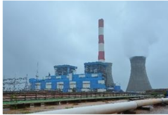
2X600MW TPP, BOILER & STG, MANGALORE, LANCO (COMPLETED)
