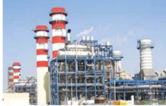
2X157 MW GT POWER PLANT, LIBYA (COMPLETED)
