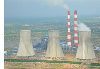
2X660 MW JTPP, BOILER,ESP & CP, JHAJJAR, STEPC (COMPLETED)
