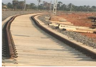
GDV-MTM 37 ,DOUBLING & ELECTRIFICATION WORKS , RVNL
