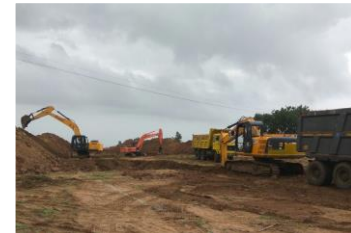
KALWESHWARAM CANAL PROJECT, 54 KM RAMAYAMPET
