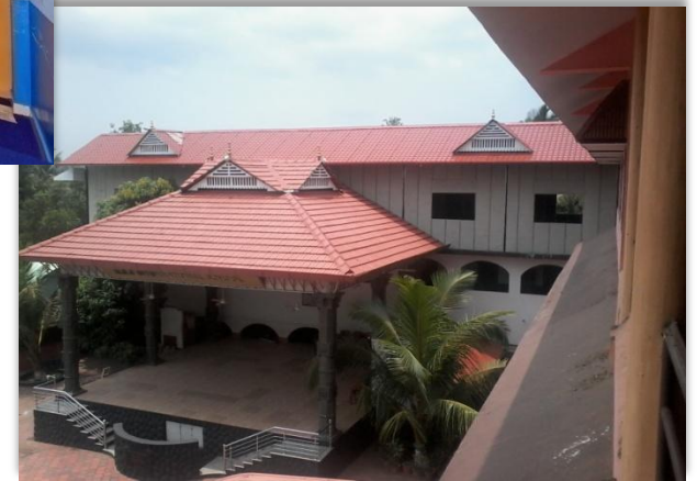
Roof Top Extension - (V-Panel )
