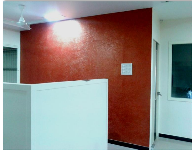
Wall Paneling - (V-Board)
